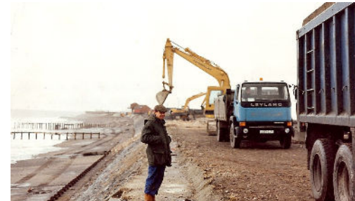
Defence repairs, Chapel St Leonards, 1970s
