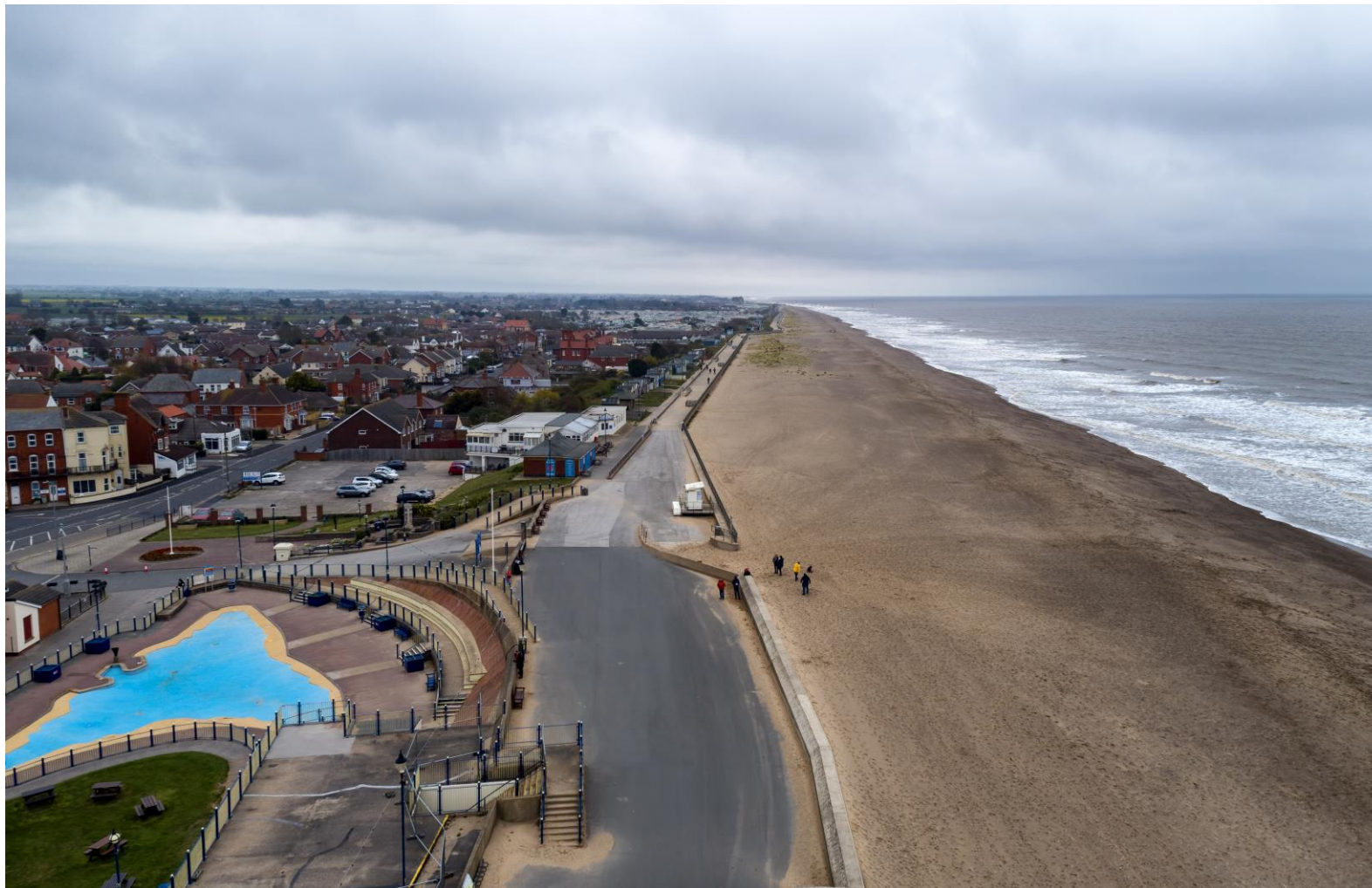
Aerial of Sutton-on-Sea coastline featuring a promenade and planted raised earth bunds in the distance.
